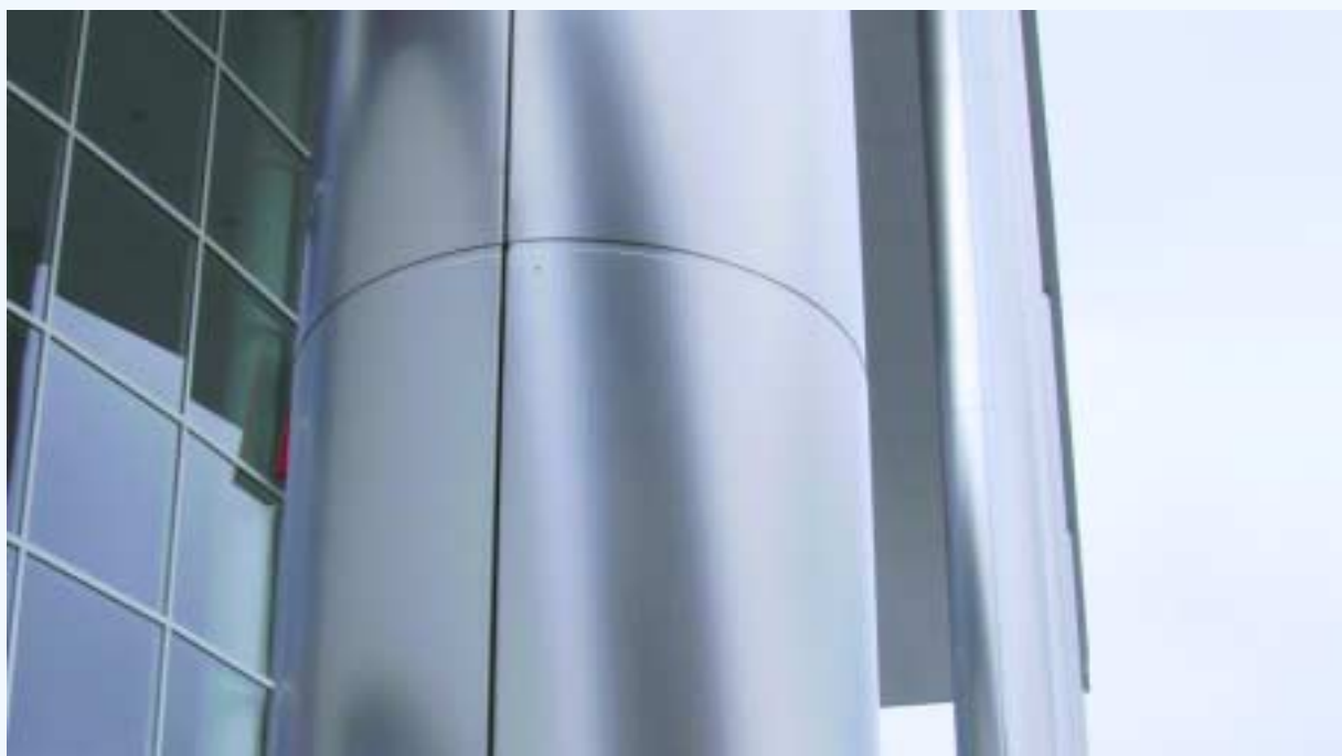
CNC-Technologie in Blech
